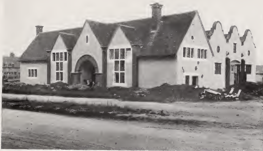
Illus. 103a.—The St. Edmundsbury Weaving Works, Letchworth. Barry Parker and Raymond Unwin, Architects.
